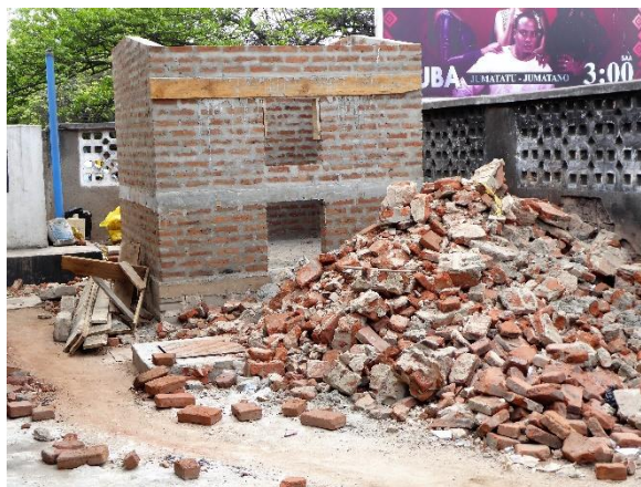
Photo 28: New incinerator under construction adjacent to the new autoclave at the Mbagala Ranji Tatu Hospital.
